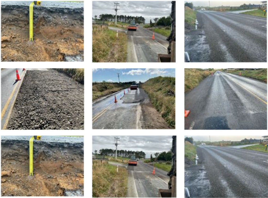
Figure 2: Progress on pavement repairs at various locations on Opunake Road
