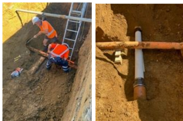
Figure 9: Council contractors relocating the 11 KV powerline and repairing the sewer pipe
