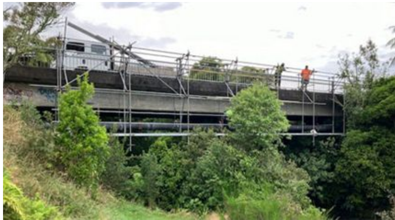
Figure 3: Swansea Road scaffolding for pipeline remediation works
