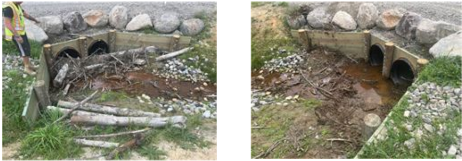
Figure 1: Blocked Drainage Repair at Puniwhakau Road- Before and After
