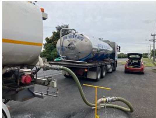
Figure 6: Temporary bulk water filling point
