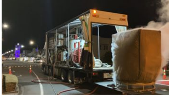
Figure 10: PVC liner being steam heated prior to insertion and expansion.
