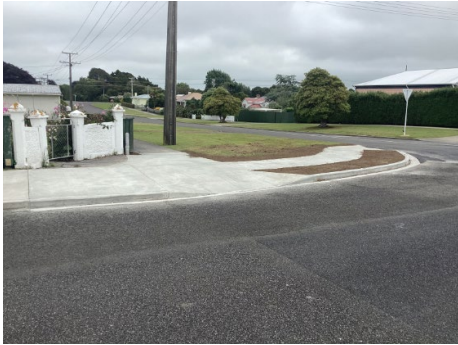
Figure 3: New footpath on the corner of Fenton Street and Cordelia Street.
