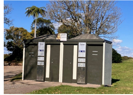
Figure 22: Exeloo Toilets (Southern End)
