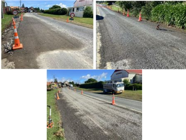
Figure 2: Pavement repairs on Cardiff Road.
