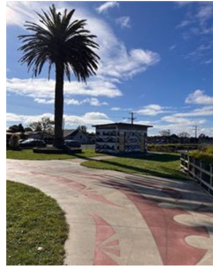
Figure 2320: Exeloo Toilets (Northern End)
