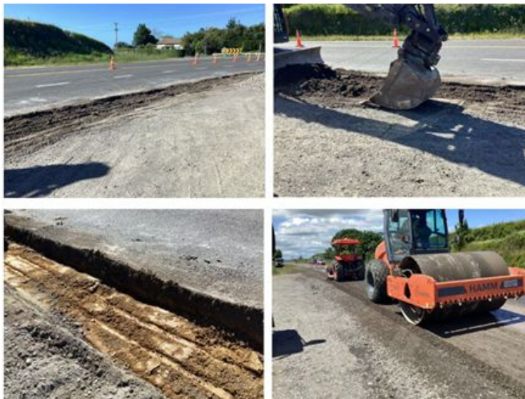
Figure 1: Pavement repairs on Opunake Road.
