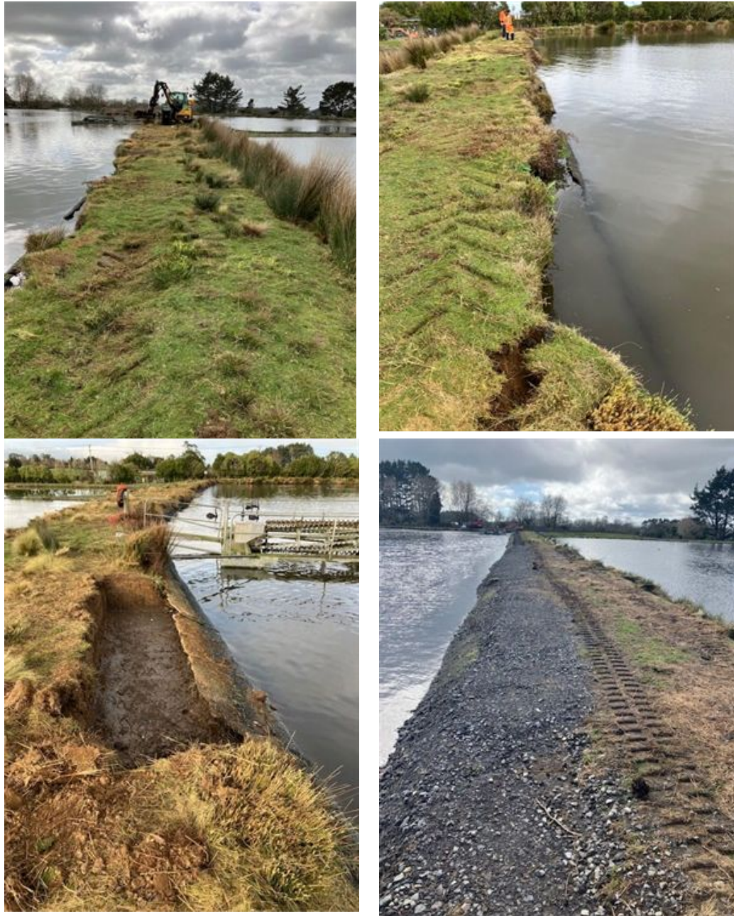
Figure 7: Wastewater pond wall stability works
