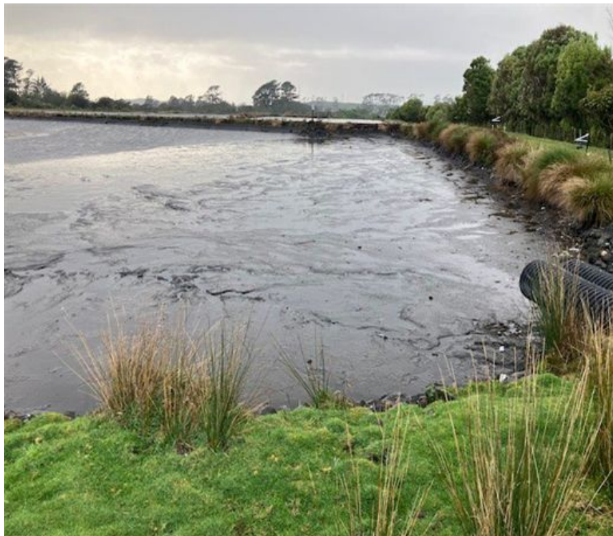
Figure 8: Wastewater treatment pond sludge buildup
