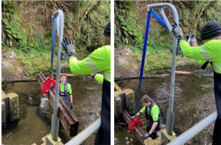
Figure 8: Konini Dam Boards Installation
