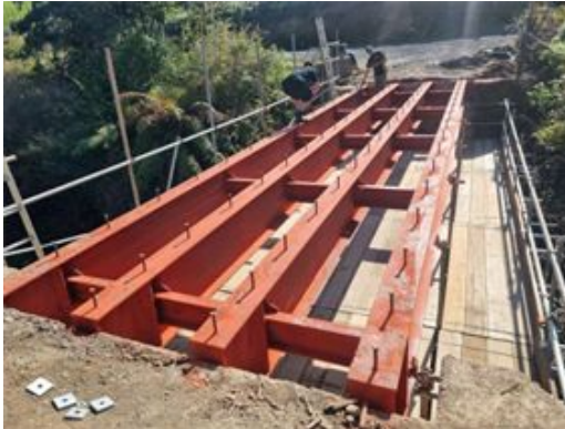
Figure 3: New Steel Beams for the Bridge.
