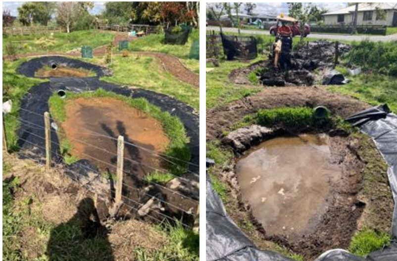
Figure 11: Private Ponds Sediment Removal Works
