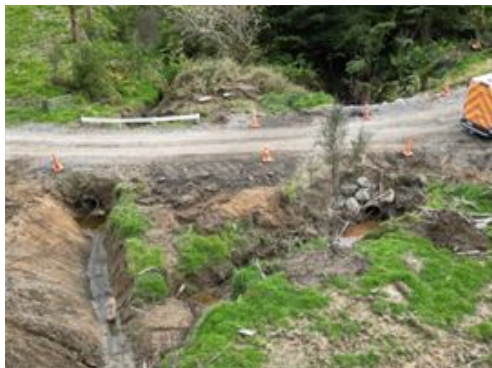
Figure 1: The existing 600mm concrete culverts once cleared of the forestry slash.
