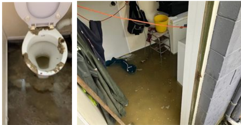
Figure 10: Sewage Overflow from Basement Toilet into Adjacent Laundry and Garage
