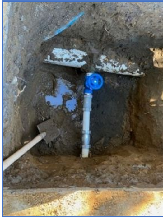
Figure 6: Eastern Valve Replacement
