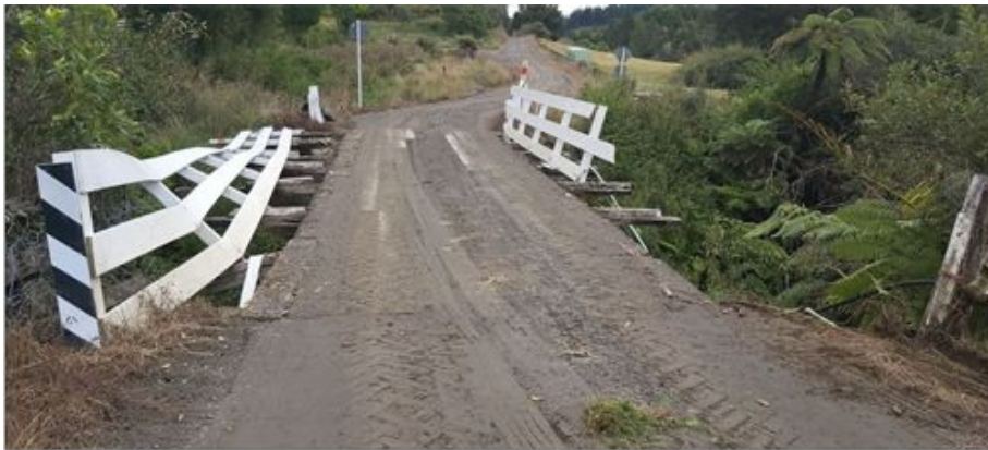
Figure 3: Damage to the temporary handrail and supporting beams.
