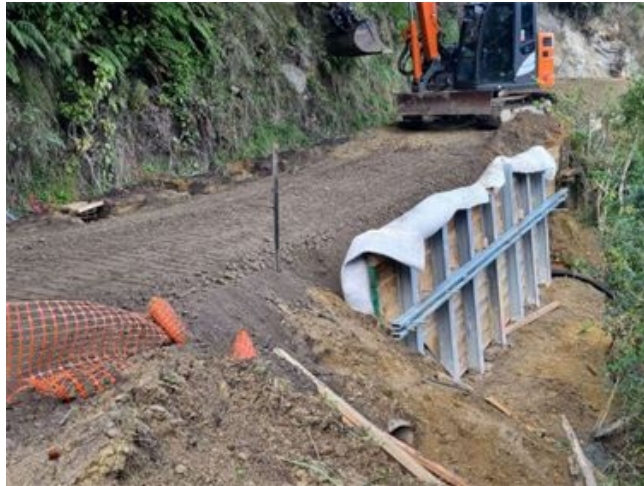
Figure 4: Extending the retaining wall on Junction Road
