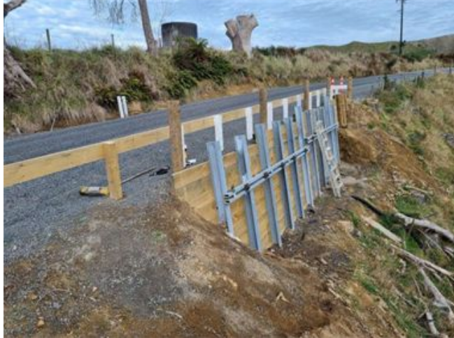
Figure 3: The completed retaining wall on Mangaotuku Road. Sight rails are being painted
