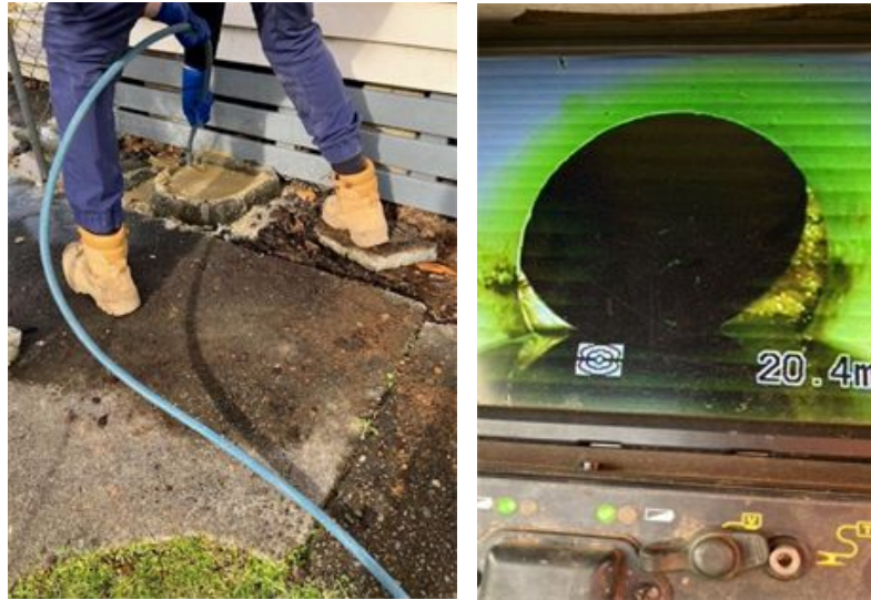
Figure 8: Gully trap overflow due to blockage Figure 9: Disjointed sewer lateral
