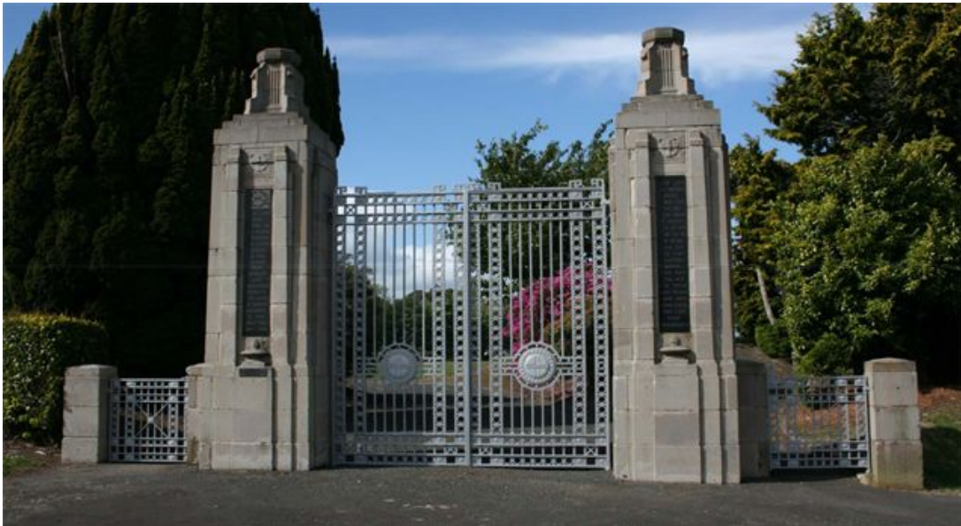
Figure 7 - Victoria Park Memorial Gates
