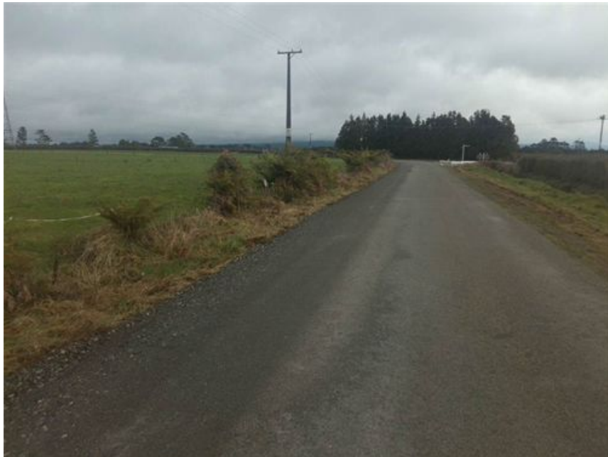
Figure 1: Shoulder widening on Radnor Road.
