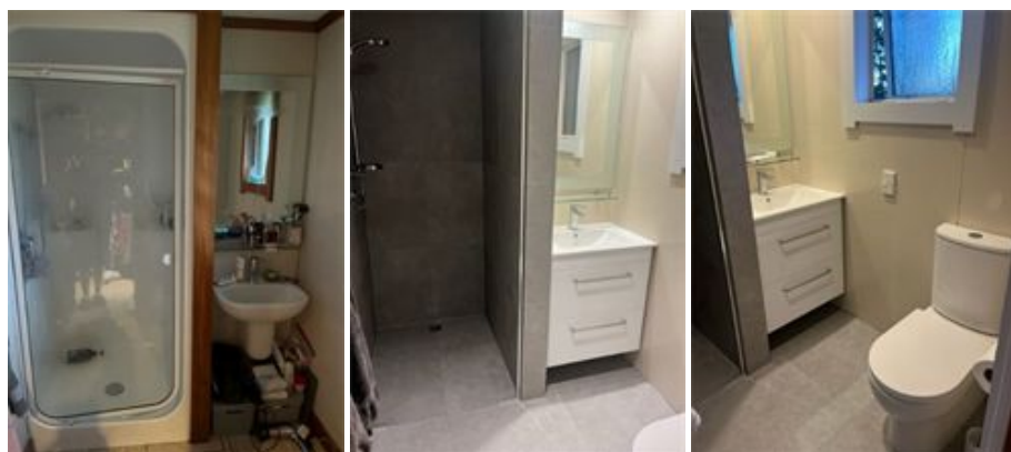
Figure 3 – Before and after photos of the farmhouse ensuite
