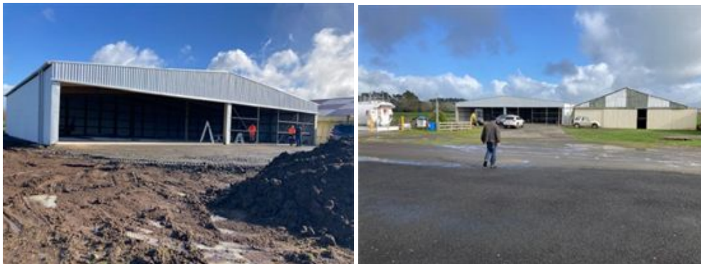
Figure 9: Progress photos of the Aero Clubs new hangar - July 2023
