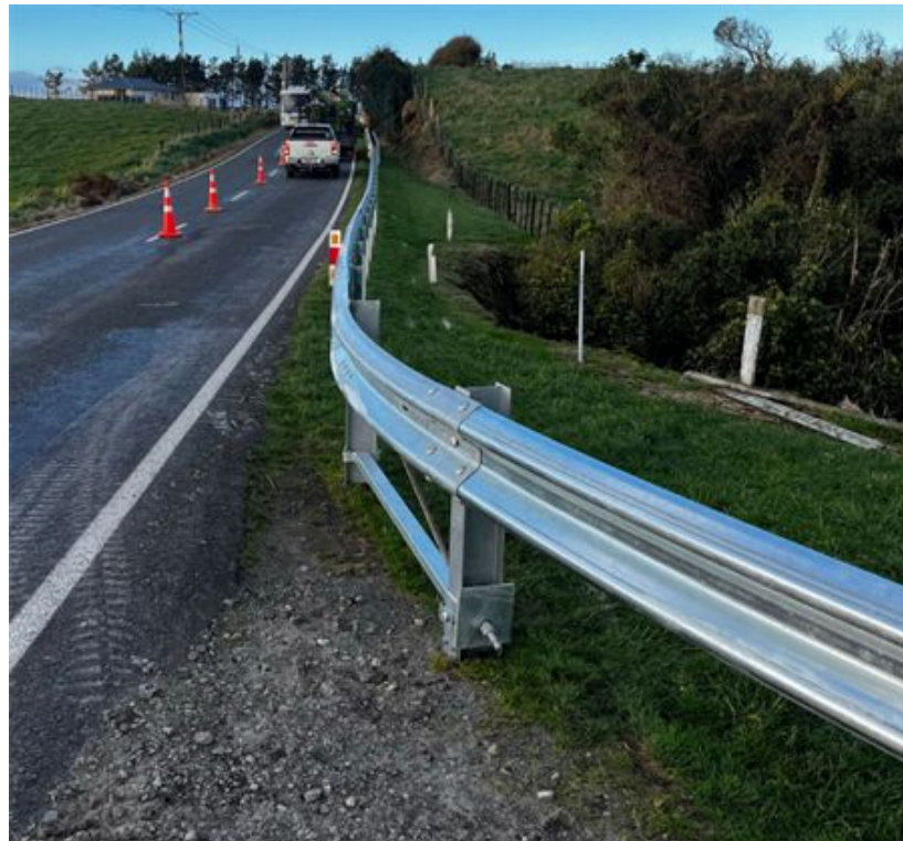
Figure 2: The Armco roadside barrier installation on Opunake Road
