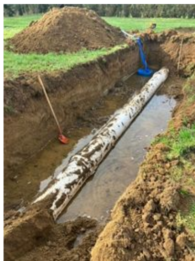
Figure 4: Broken 375 mm PVC trunkmain
