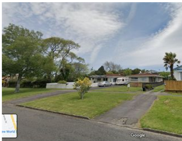
Figure 4: Option 3 - Widening the existing footpath will steepen the gradient of these driveways.
