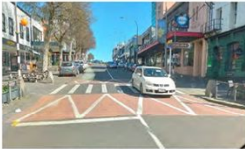
TYPICAL RAISED PLATFORM WITH CROSSING
