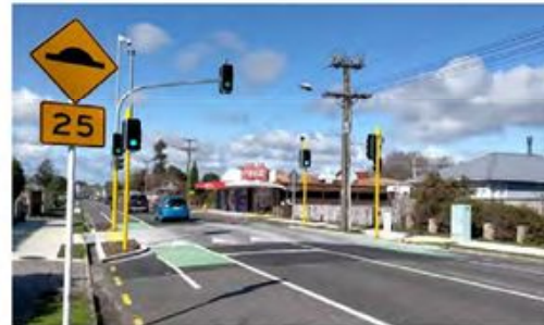
TYPICAL RAISED PLATFORM WITH TRAFFIC CONTROL
