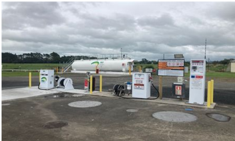
Figure 3: Completion Photo of RD Petroleum Jet A1 Fuel Tank and Dispenser
