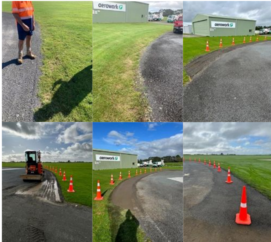
Turning Bay extension Progress photos
