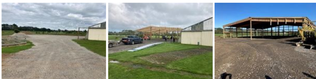
Figure 1 Aero Club New Hangar progress photos
