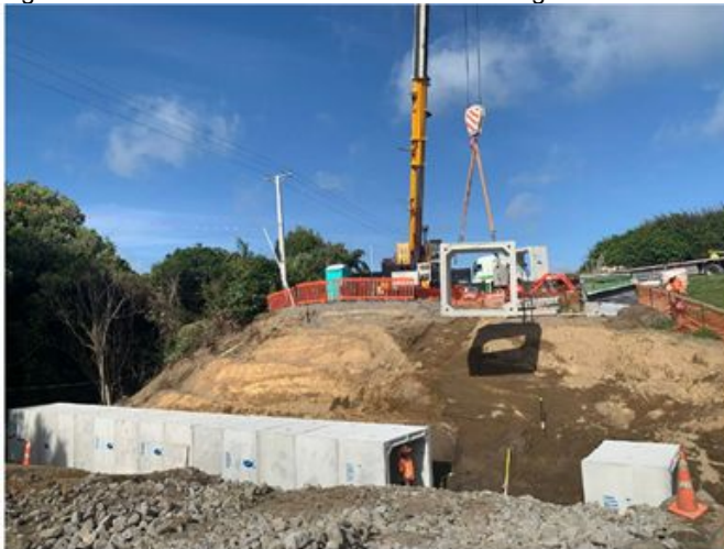
Figure 2: Monmouth Road Steel Culvert - Concrete box units being lifted into place.
