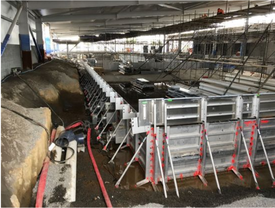
Figure 8: Lane pool side panels almost ready for back-filling
