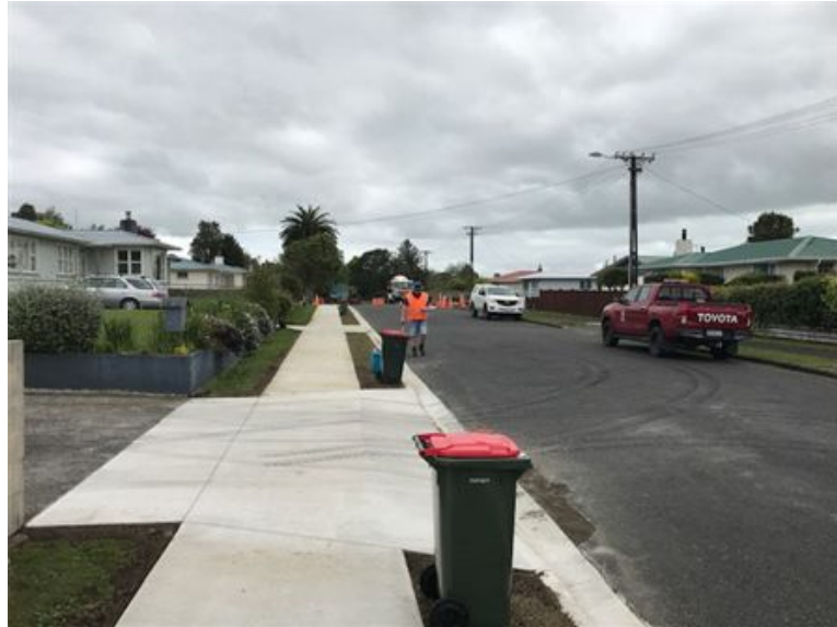
Figure 4: One side of Fabian Street with new kerb, channel and footpath
