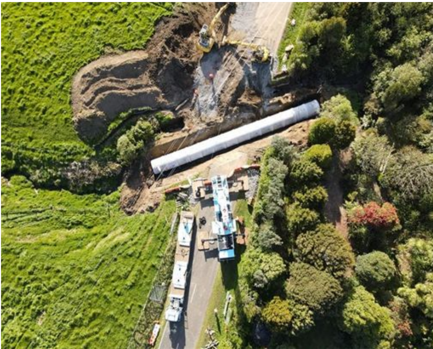
Figure 2: New culvert pipes placed in the trench across Manaia Road
