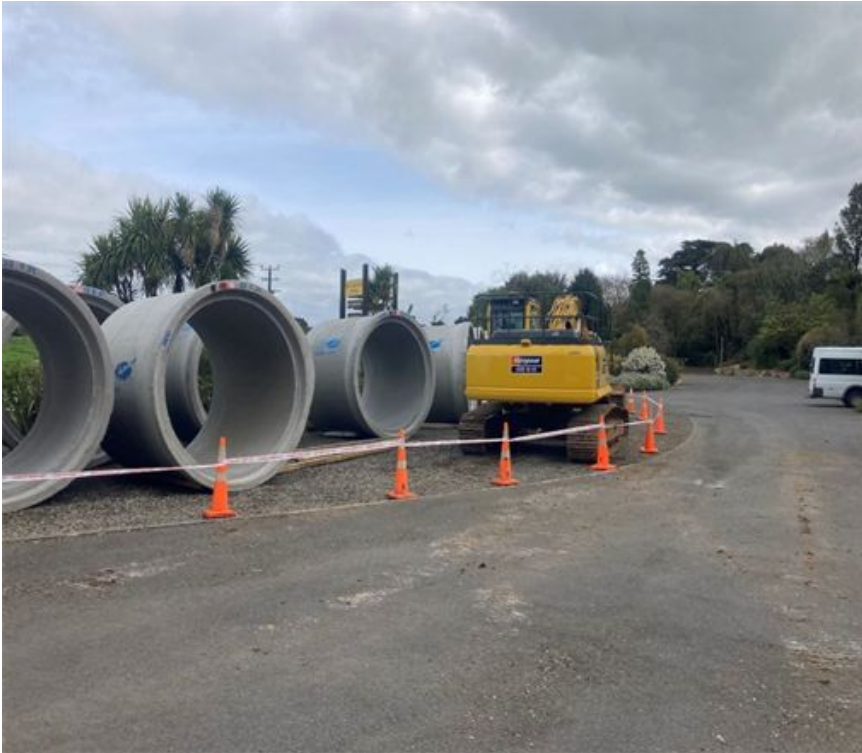
Figure 1: New concrete culvert pipes stored in the carpark of Hollard Gardens
