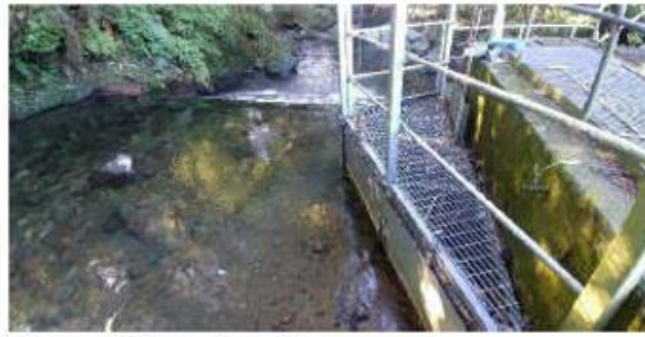
Patea River intake structure
