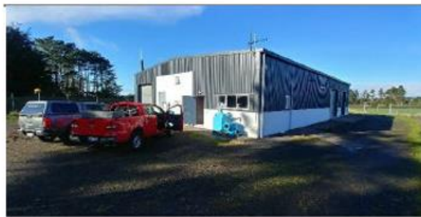
Water Treatment Plant main building
