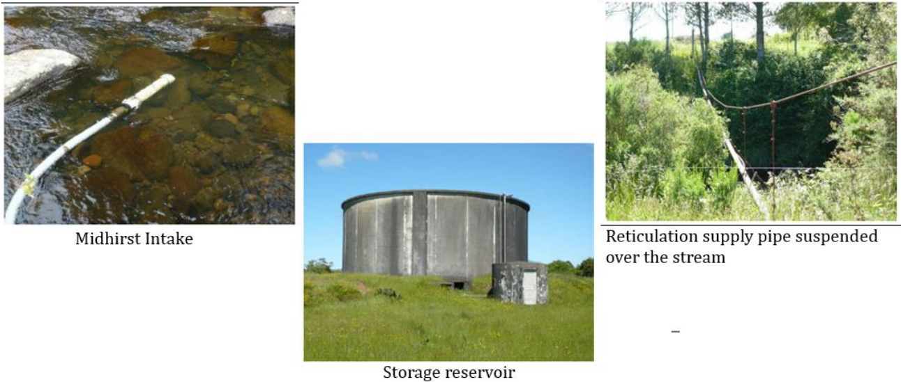
Figure 13 - Midhirst Water Plant Photos
