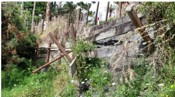
Wall #382: Mangaowata Road
