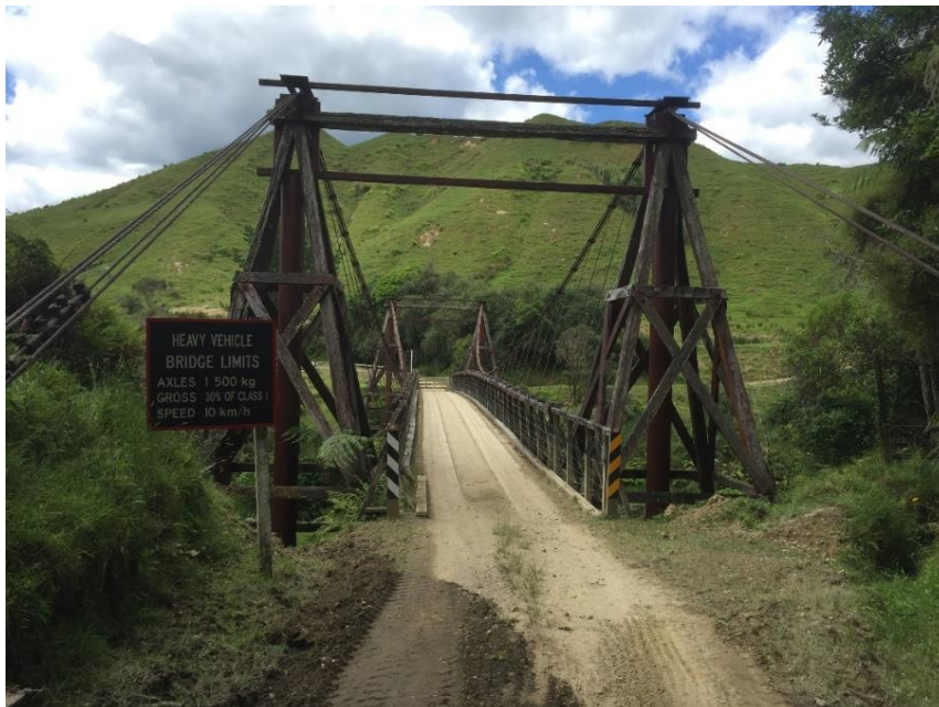
Figure 33 - Lower Kohuratahi Road Bridge
