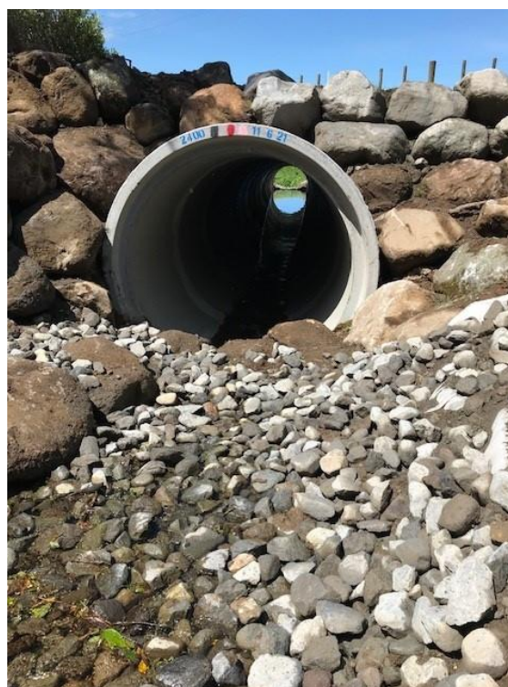
Newly installed culvert
