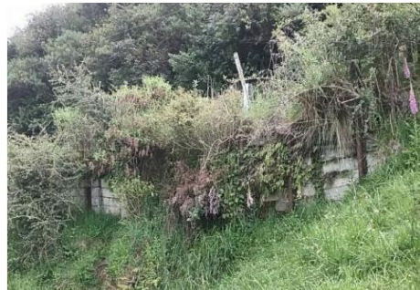
Wall number 227: Mangaehu Road
