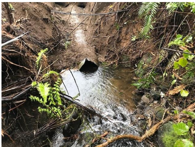
Existing culvert that was removed
