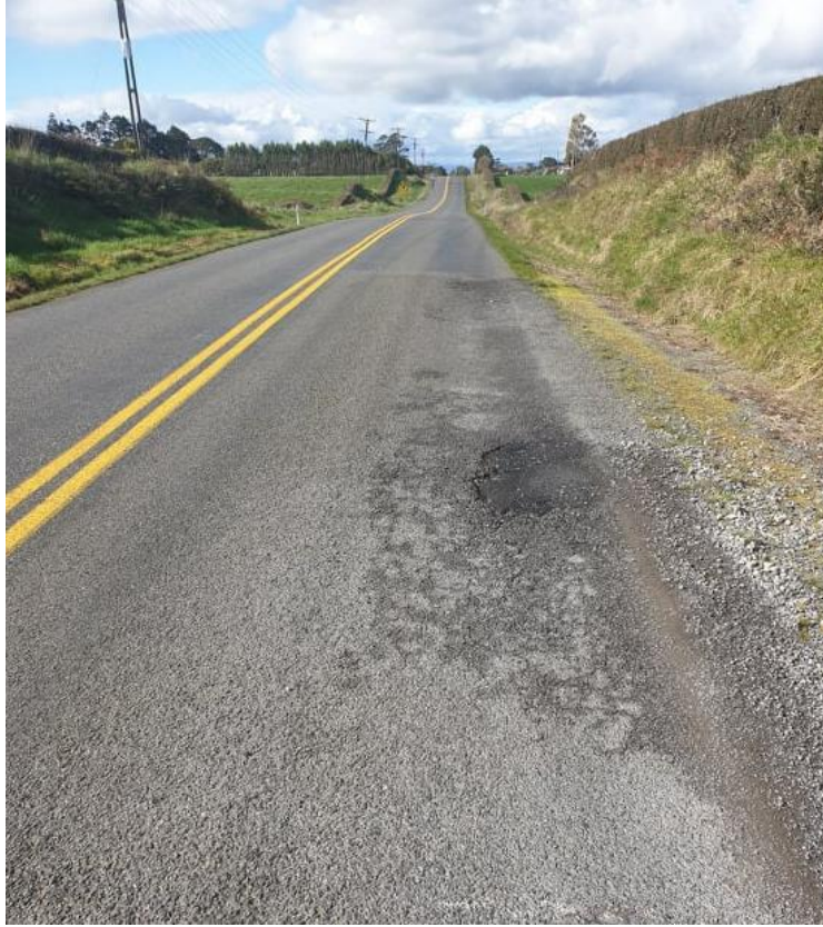
Figure 49 - Photo of Opunake Road a HMPV Route.
