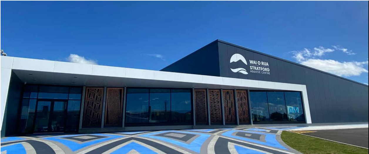
Figure 9 – Wai o Rua -Stratford Aquatic Centre
