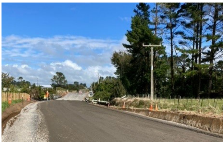
Cardiff Road realignment project completed.
