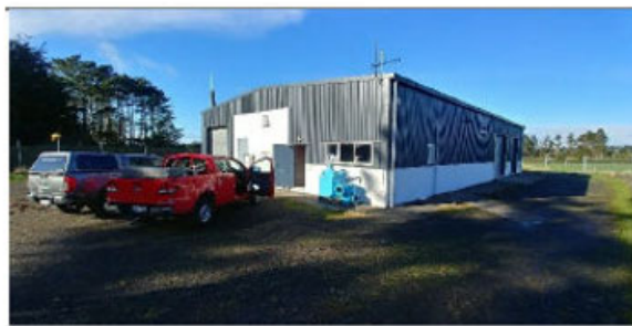
Water Treatment Plant main building
